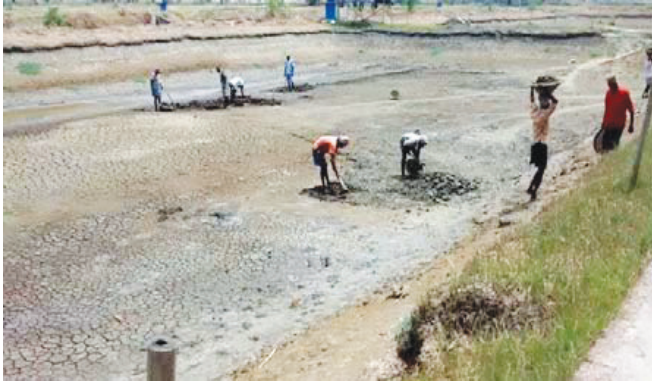
Pond bottom soil removal
