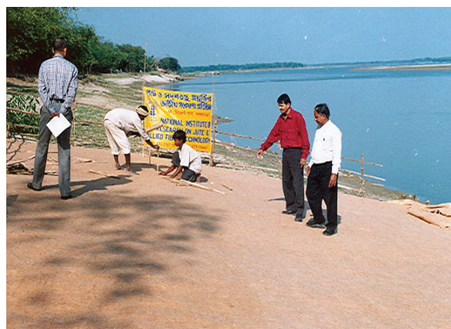
Fig. 2. Levelling of land surface before laying jute geo-textile
