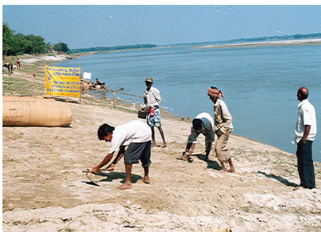
Fig. 1. Laying of jute geo-textile mulches on the river bank
